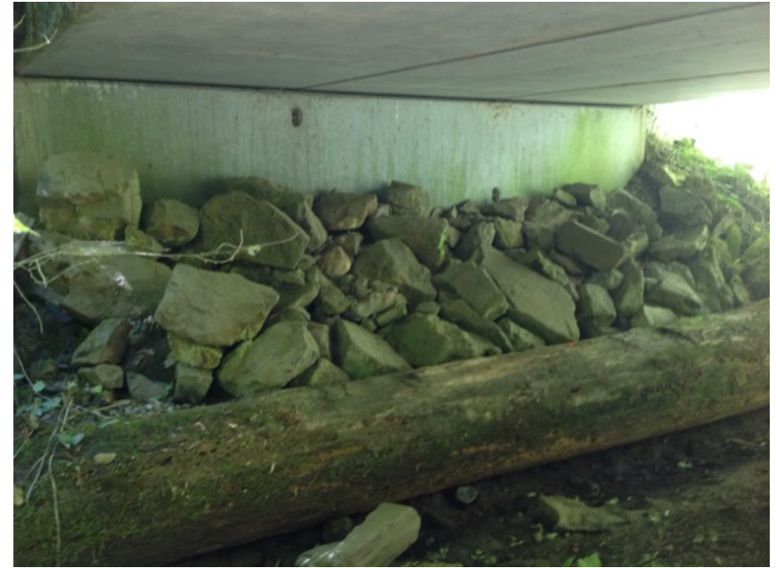
Left Bank Abutment when facing downstream
