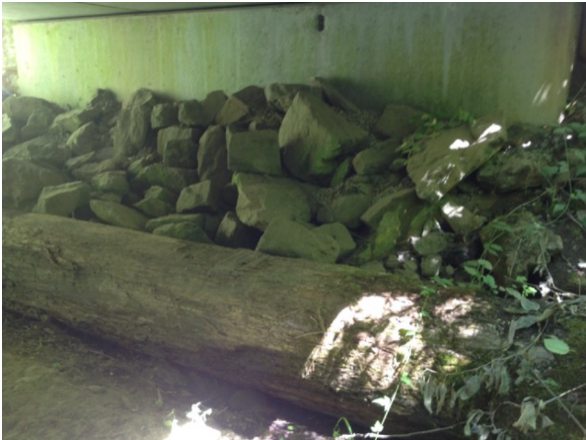
Right Bank Abutment when facing downstream
